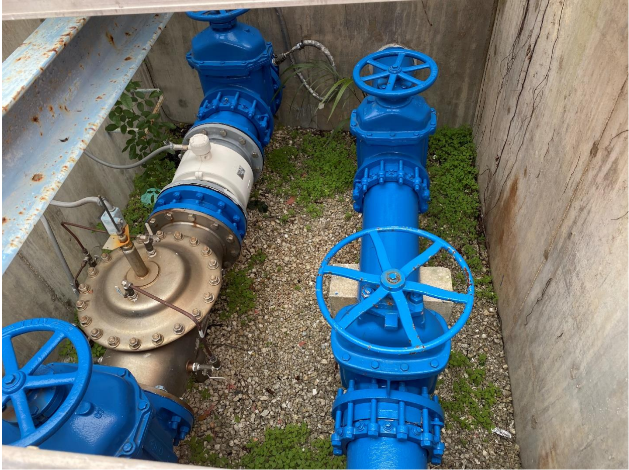
Figure 3. Fill and Flow Meter Vault
